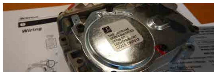
Figure 13.k Conversion label on valve
