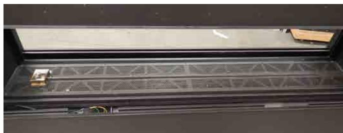
Figure 25.g Insert pilot cover/door/screen
