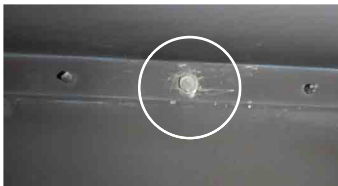
Figure 26. Remove the existing screws
