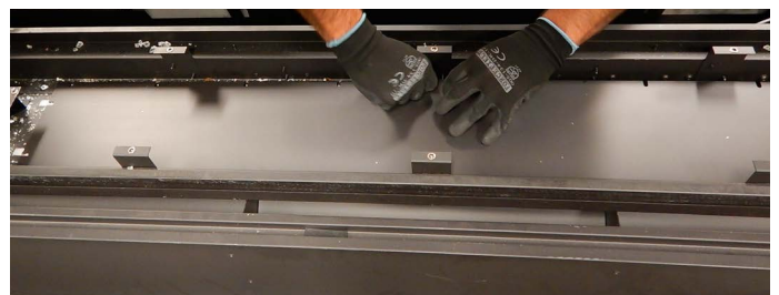
Figure 12.g Removing metal plate
