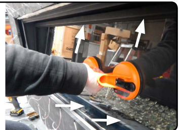
Figure 21.b Installing the door
