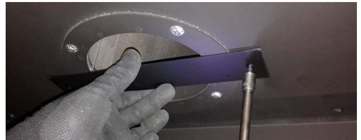
Figure 8.b.c Restrictor plate Installation
