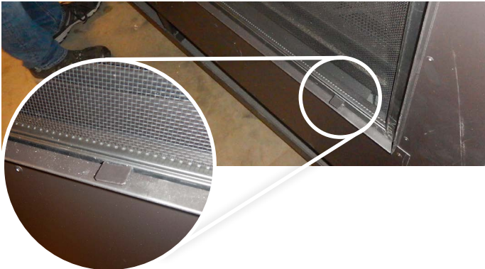
Figure 20. Locate the three tabs at the base of the screen
