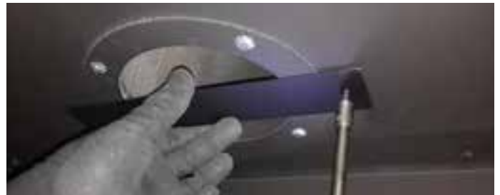
Figure 8.b.c Restrictor plate Installation
