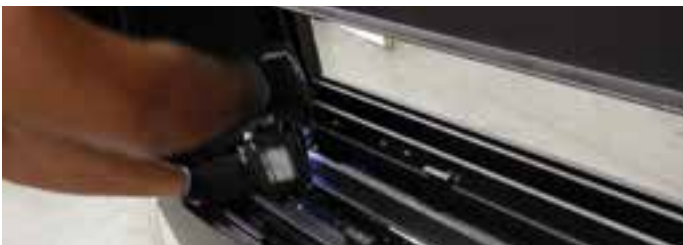
Figure 12.d Removing the Burner screws
