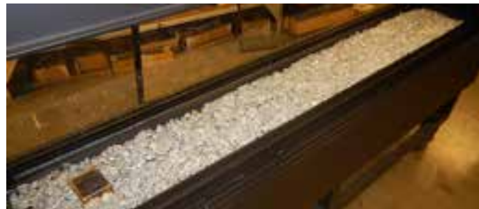
Figure 22.b Completed glass Firestone installation.
