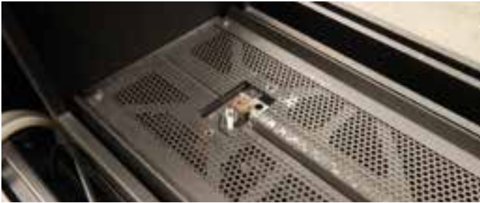
Figure 12.a Removal of the pilot cover
