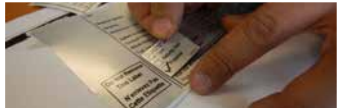
Figure 13.j Conversion label on rating plate label
