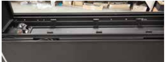
Figure 12.e Removing the Burner
