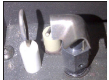
Figure 23: Proper Pilot Position
