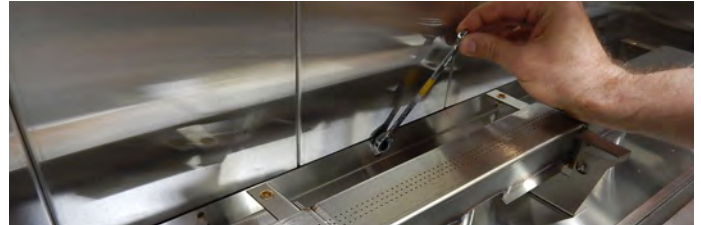
Figure 52 Loosening air baffle bolts
