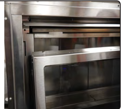
Figure 63 Completing removal of the door
