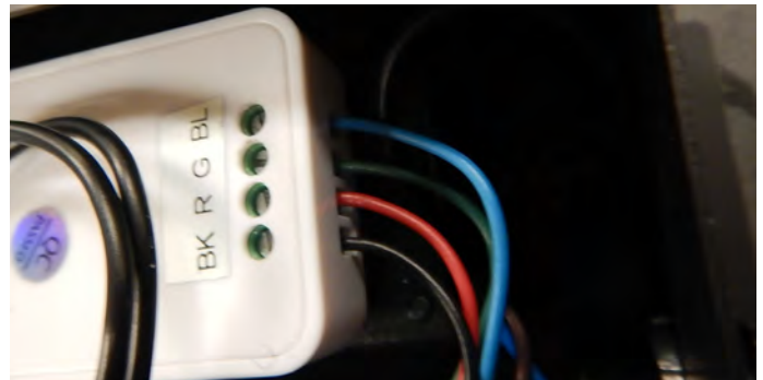
Figure 48 Wiring the LED receiver
