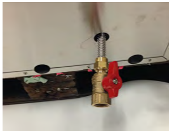
Figure 12 Gas connection
