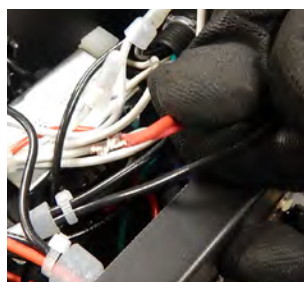
Figure 38 Connecting the wires
