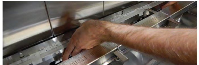
Figure 54 Installing LED air baffle
