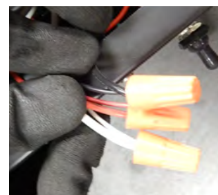
Figure 39 Connecting the wires
