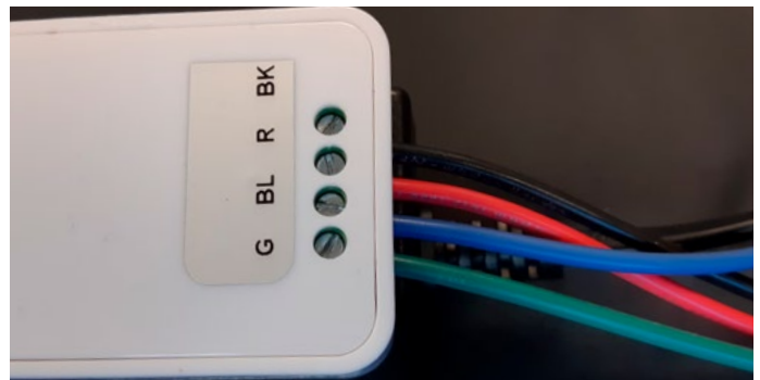
Figure 48 Wiring the LED receiver
