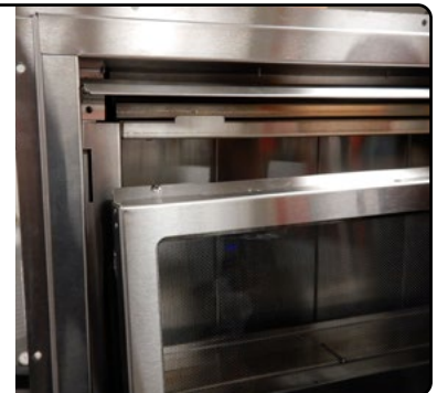
Figure 64 Completing removal of the door
