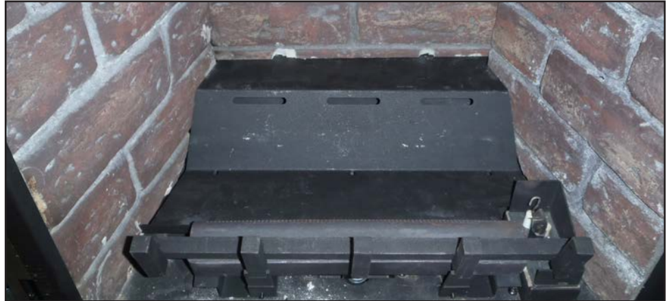
Figure 50. Empty firebox with grate and locator pins.
