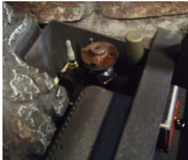
Figure 15. Pilot assembly beside the burner.
