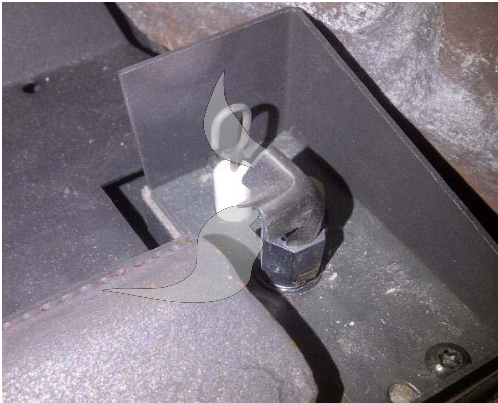
Figure 23. Correct Burner & Pilot Shield Placement (Q1 IPI model shown but similar to Q2 IPI model)
