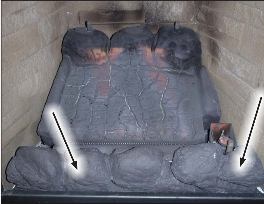
Figure 58. Second Stage Coal Set Installation.
