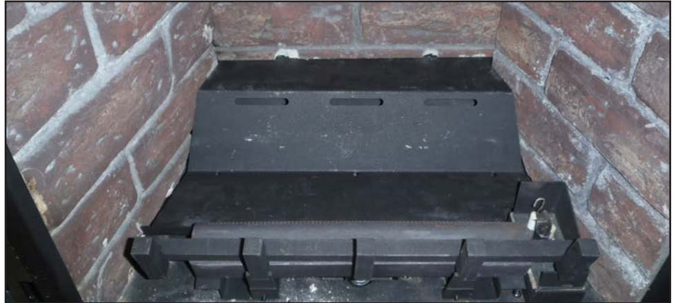
Figure 56. Empty firebox with grate and locator pins.
