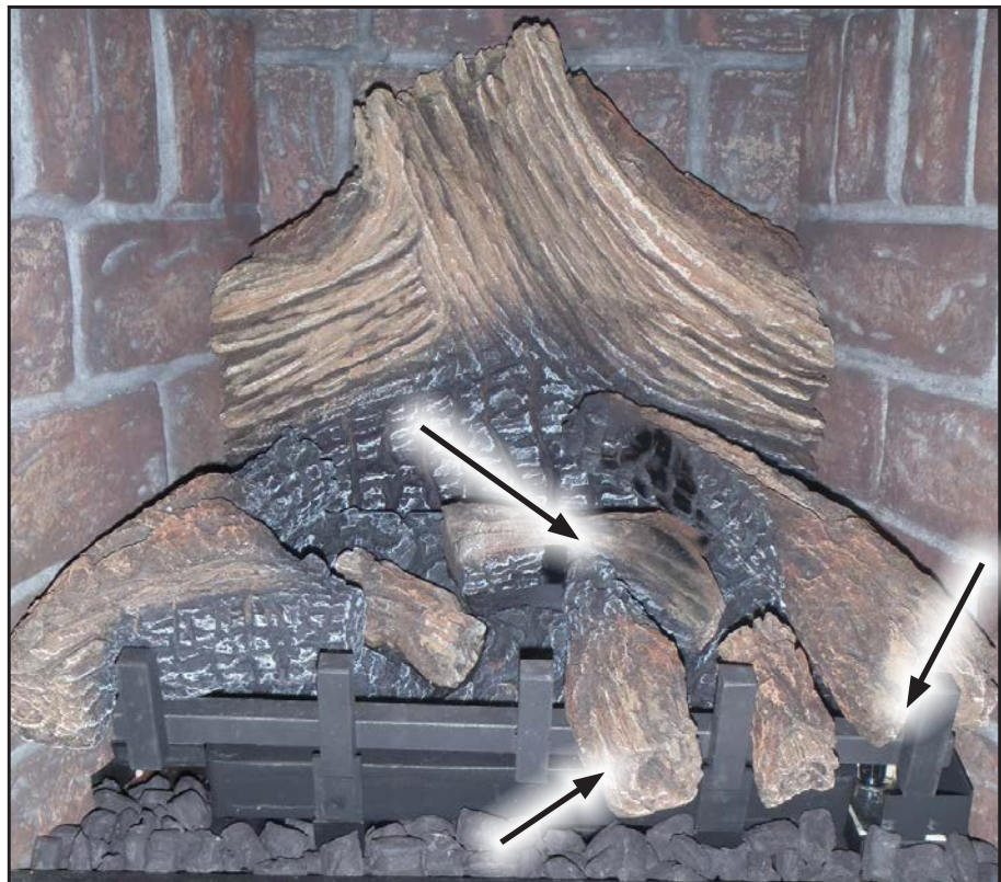
Figure 60. Fourth Stage Log Set Installation.
