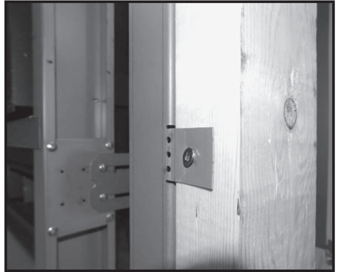
Figure 16: Attach tab to wood framing.
