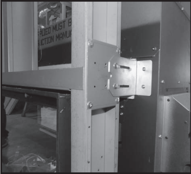
Figure 15: Framing bracket positioning.
