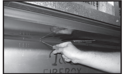
Figure 38: Securing top porcelain panel.
