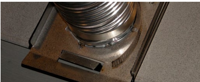
Figure 3.2 Vent Slide plate
