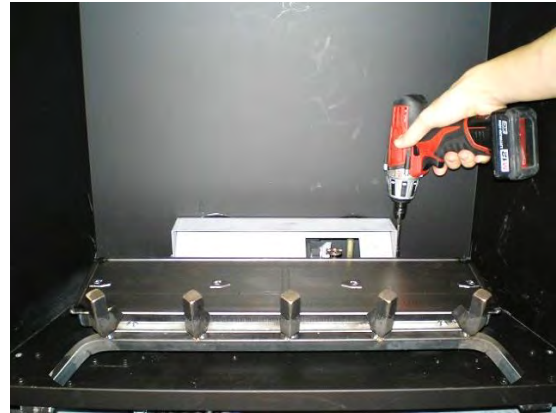
Step One: Remove Log Holder.
