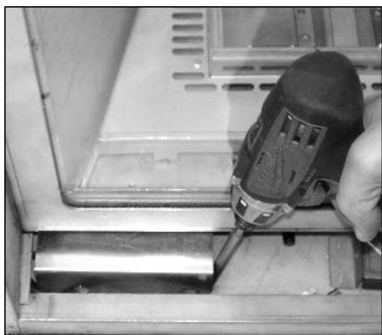
Power Vent Control Module Mounted inside fireplace.
