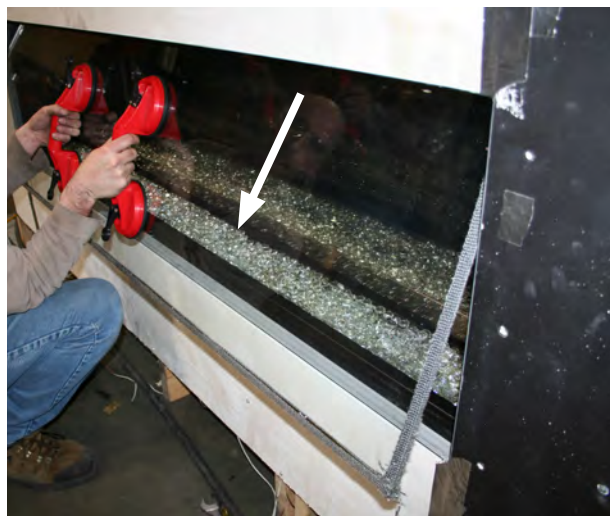
Figure 2 Sec.8 Window Removal (using glass lifting tools).
