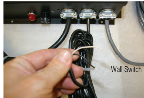
Figure 4 Sec.5 (Wall Switch Wire connection)
