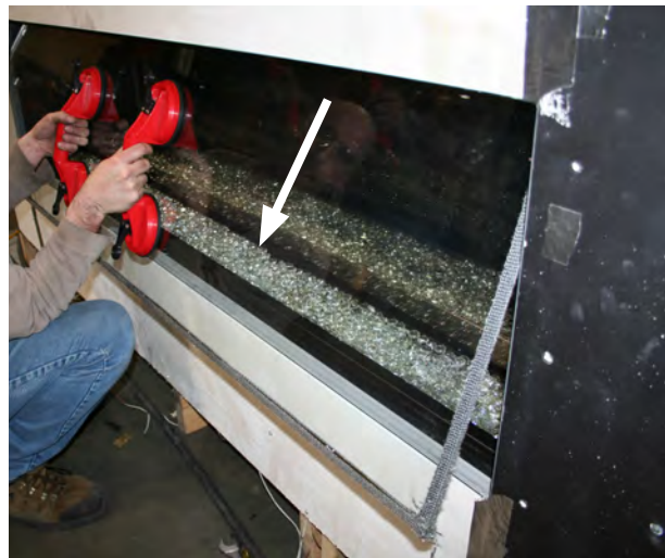
Figure 2 Sec.8 Window Removal (using glass lifting tools).
