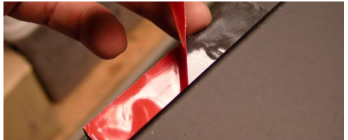
Figure 5.12b Peeling self-adhesive tape
