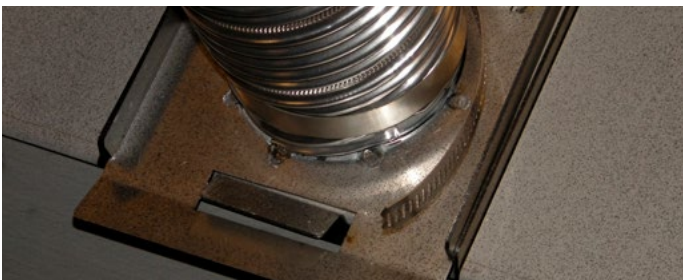
Figure 3.2 Vent Slide plate
