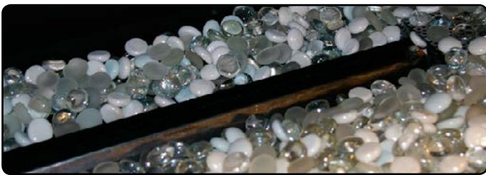
Figure 21. spreading out firestones
