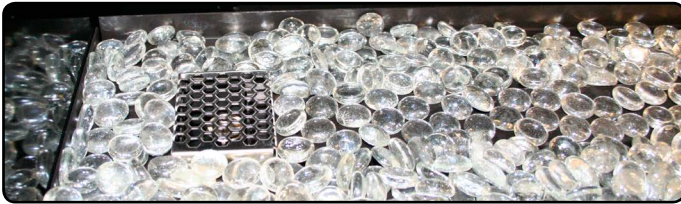
Figure 21.b Completed firestone installation
