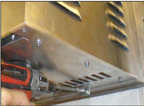
Loosen screw at bottom of Power Vent
