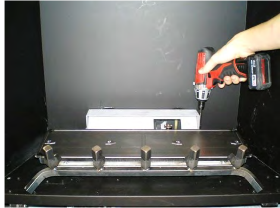
Step One: Remove Log Holder.
