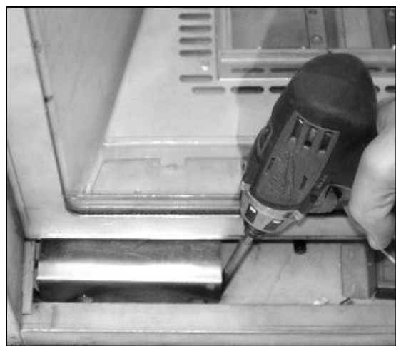
Power Vent Control Module Mounted inside fireplace.
