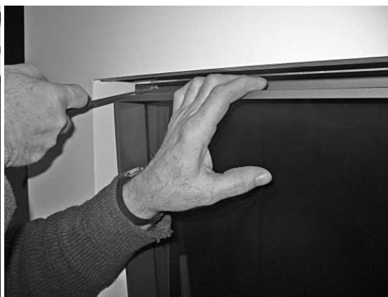
- Use the hook supplied (see photo) for opening the frame and the glass.
