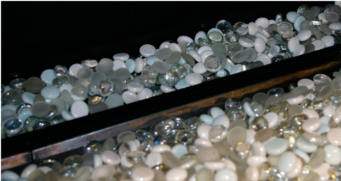
Figure 26. Completed firestone installation. Second Gen burner shown.
