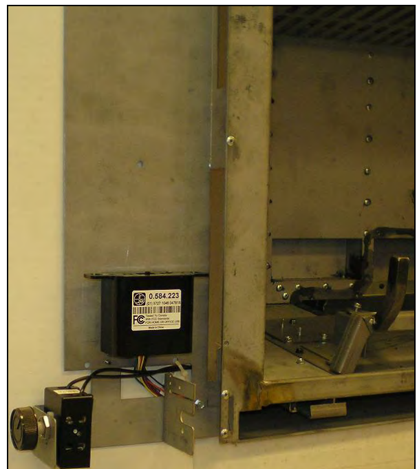
Components Out Remote Receiver Location.
