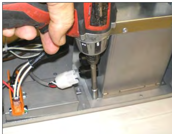
Reposition Lamp Transformer housing. Install Power Vent Control Module as shown.
