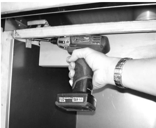
Step Four: Fix Side Liners in place using Liner Retainer Clips to replace Brick Clips.
