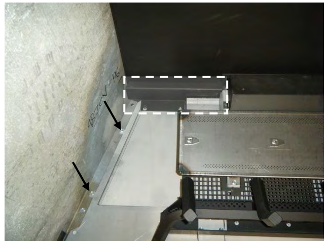
Step Five: Reinstall Liner Supports and Screws.
