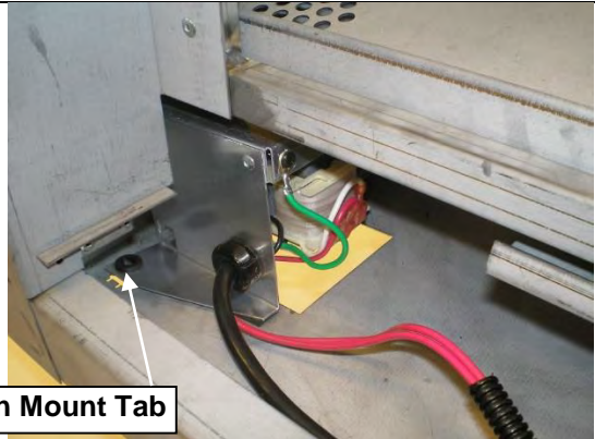
Set fan onto Mount Tabs inside fireplace.
