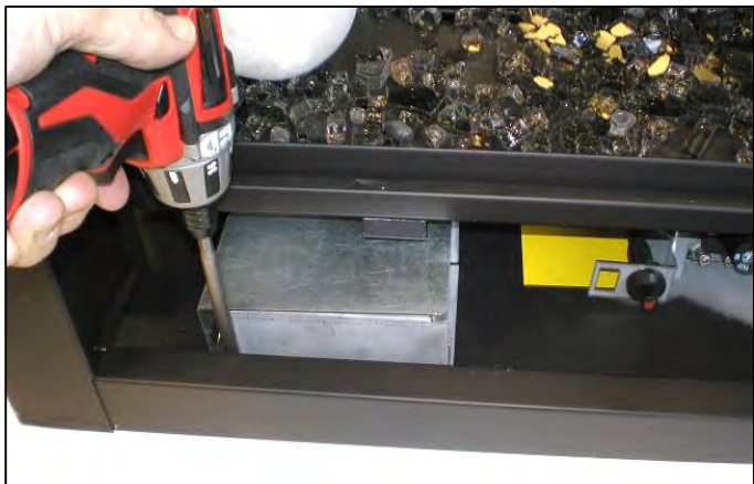
Power Vent Control Module Mounted inside fireplace.
