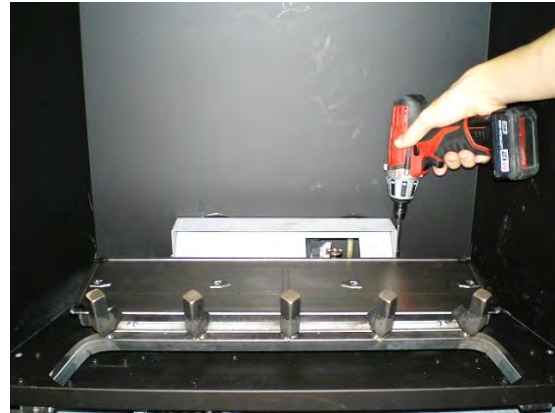
Step One: Remove Log Holder.
