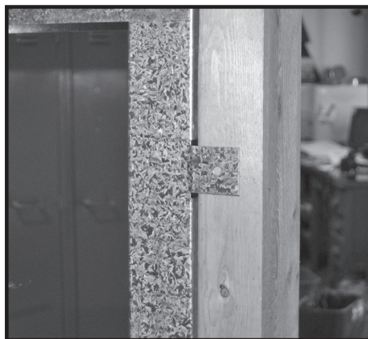
Figure 19: Attaching metal tab to frame
