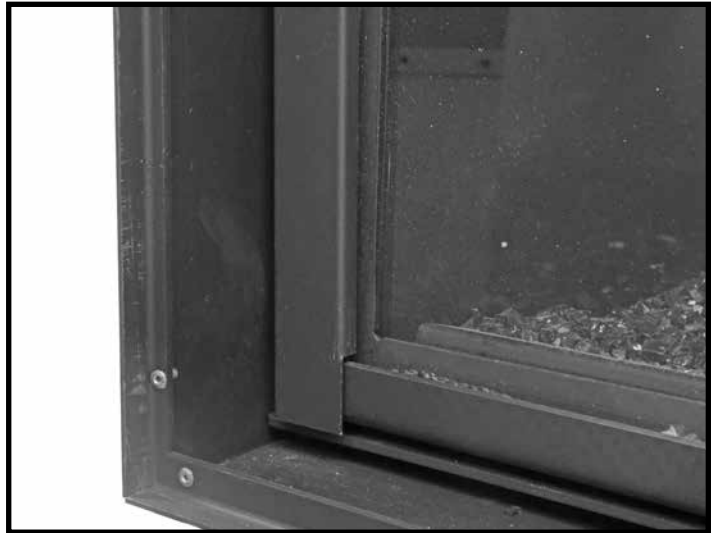
Figure 52: Side trim in place.
