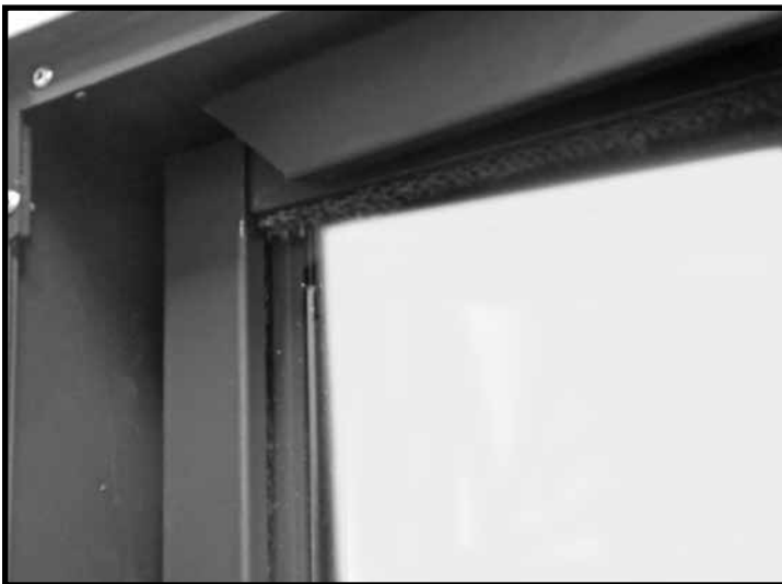
Figure 53: Installing top trim.
