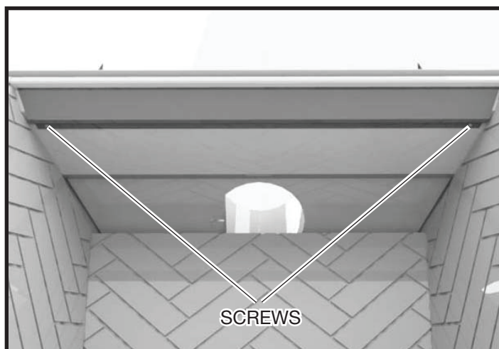
Figure 52: Side panel retainer location.
