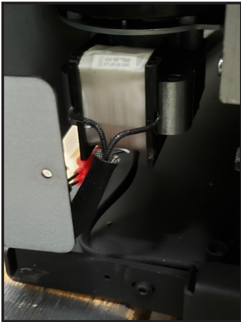
Figure 14: Wire Location LHS.
