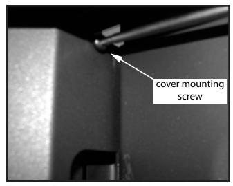
Figure 11: Front cover screw location.
