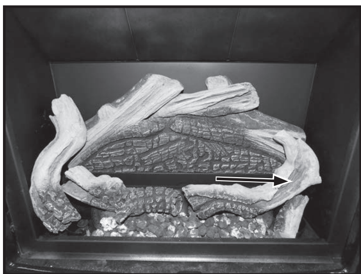
Figure 48: 5th log placement.
