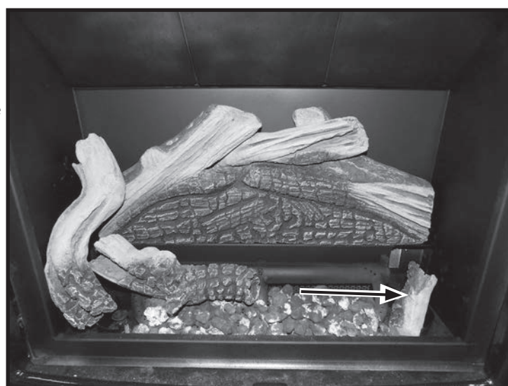
Figure 47: 4th log placement.
