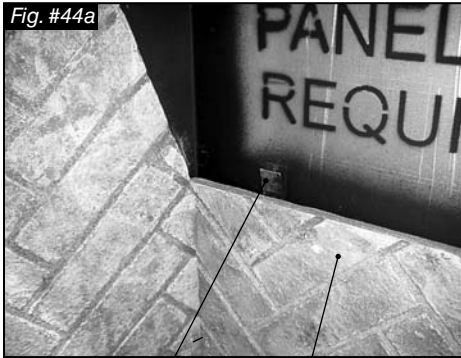
ADJUSTABLE "V" BRACKET REAR LOWER PANEL
