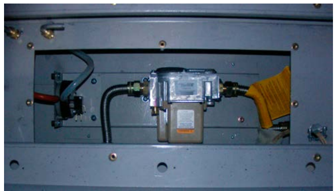
Figure 36g. Gas Valve and Pressure Sensor
