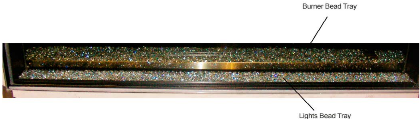
Figure 31b. Completed firestone installation
