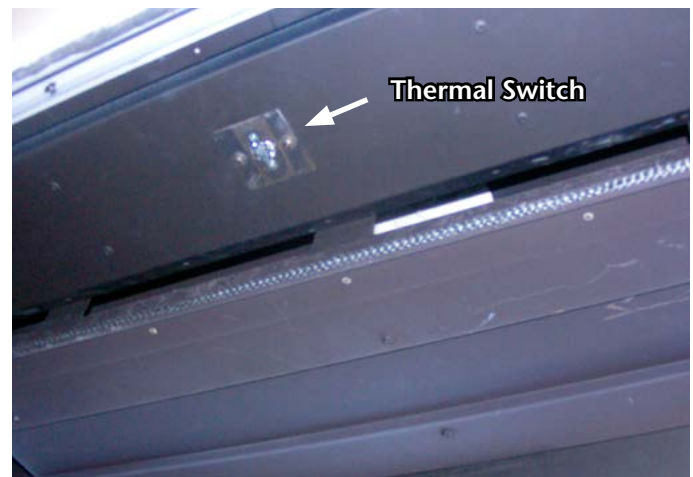
Figure 34. Thermal Switch Location
