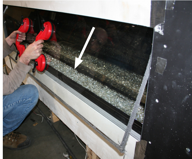
Figure 21b. Window Removal (using glass lifting tools).
