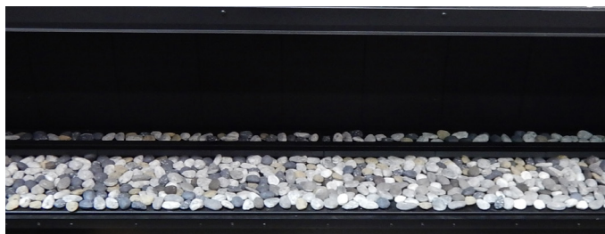
Figure 22b. Completed Speckled Stone installation.
