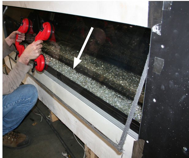
Figure 21b. Window Removal (using glass lifting tools).
