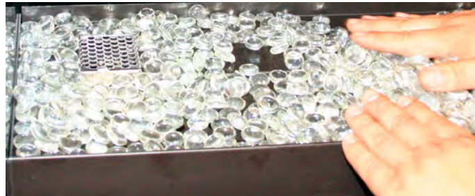
Figure 24b. Installation of the firestones. (Ensure ONLY one layer of firestones cover the surface).
