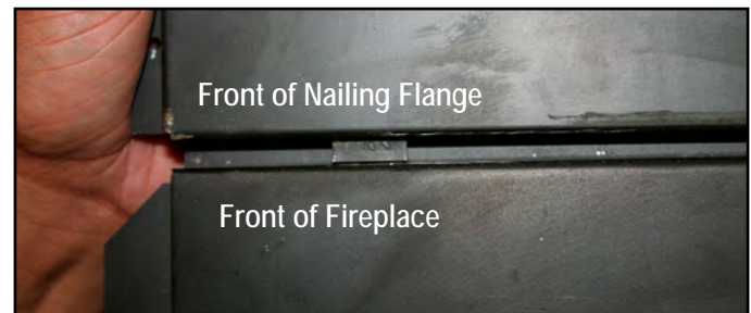
Figure 7b. Insert folded tabs into slots above the front of the fireplace
