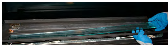
Figure 26a Place the up-lighting glass in the burner tray.
