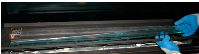
Figure 30. Remove the up-lighting glass from the burner tray.
