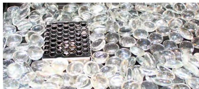
Figure 26e. Completed firestone installation. (Note: DO NOT place ANY firestones on top of the pilot cover).
