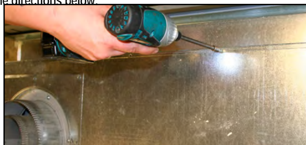
Figure 7. Remove screws from top of the unit
