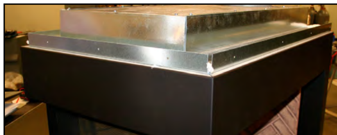
Figure 7c. Finished removing Nailing Flange extension.
