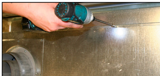
Figure 7. Remove screws from top of the unit
