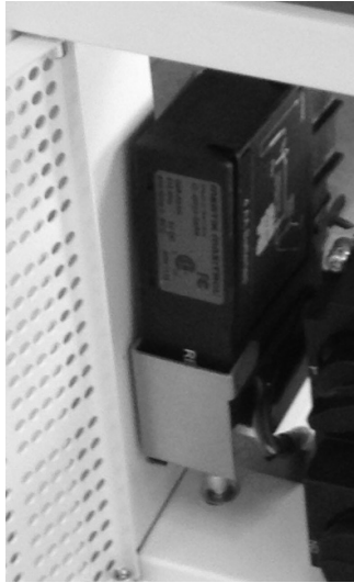
Figure 28 Receiver in Wall Access Door
