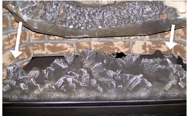
Figure 18 Sec.9 Log 1 Installation
