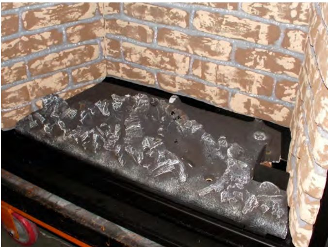
Figure 31 Sec.10 Log burner correctly installed
