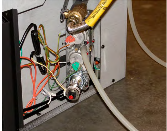
Figure 29 Sec.6 Shown on manifold tap
