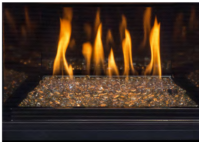
Figure 91 Sec.4 Completed firestone installation
