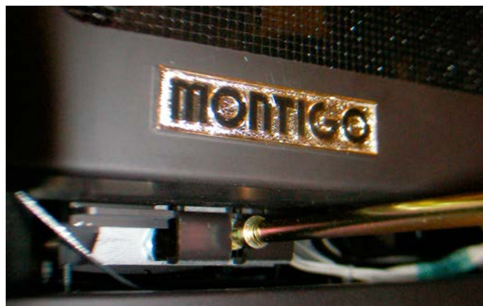
Figure 2 Sec.5 Engaging the Door Tool into the Door Retainer
