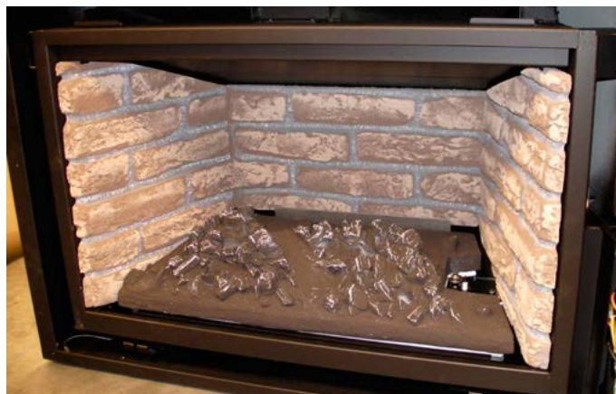
Figure 6 Sec.9 Completed brick installation
