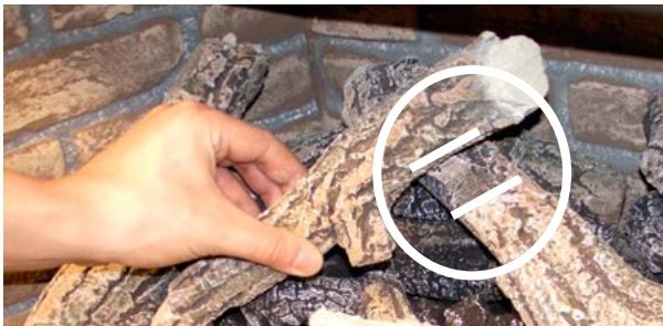
Figure 32 Sec.9 Log 8 installation detail
